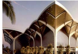
Haramain High Speed Railway Project Mecca & Médina Stations / Saudi Arabia
