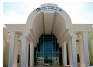
Qatar Academy Doha / Qatar
