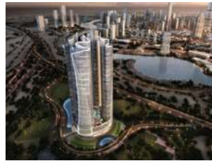
Damac Towers by Paramount Dubai/ E.A.U
