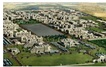
Internal Security Force (ISF) Camp Doha / Qatar
