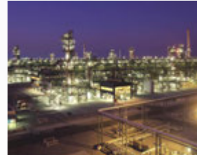
GASCO HABSHAN PROJECT (United Arab Emirates)
