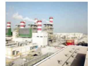
UMM AL HOUL POWER PLANT (Qatar)
