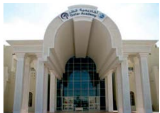
Qatar Academy Doha / Qatar
